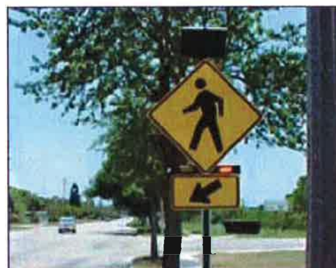
Figure 2: Activated, solar-powered, roadside RRFB at a mid-block crosswalk
