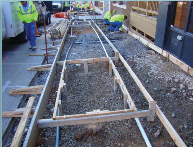
CENTER ST. during reconstruction
