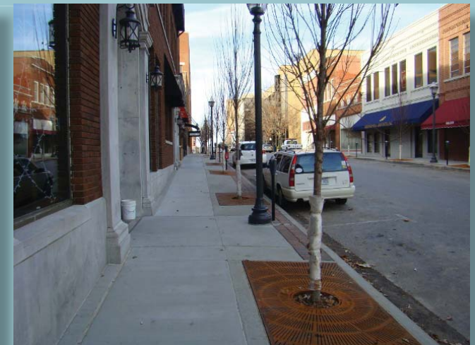
CENTER ST. after reconstruction
