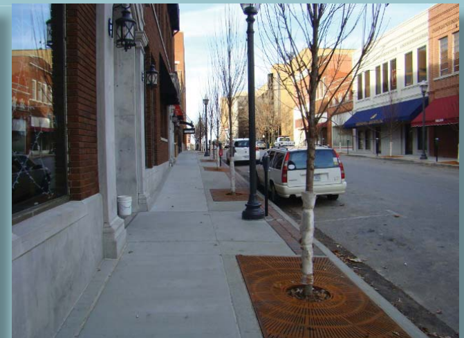
CENTER ST. after reconstruction
