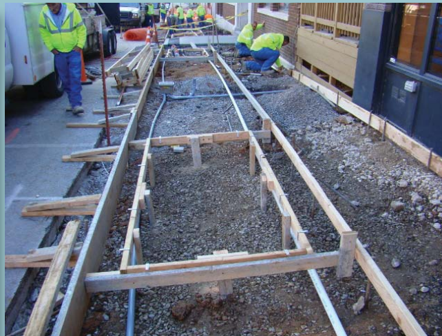
CENTER ST. during reconstruction
