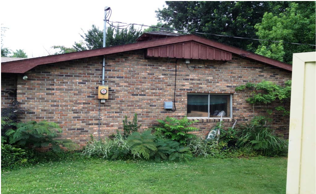
NORTHEASTERN ELEVATION OF 2634 OLD WIRE ROAD LOOKING SOUTHWESTERLY
