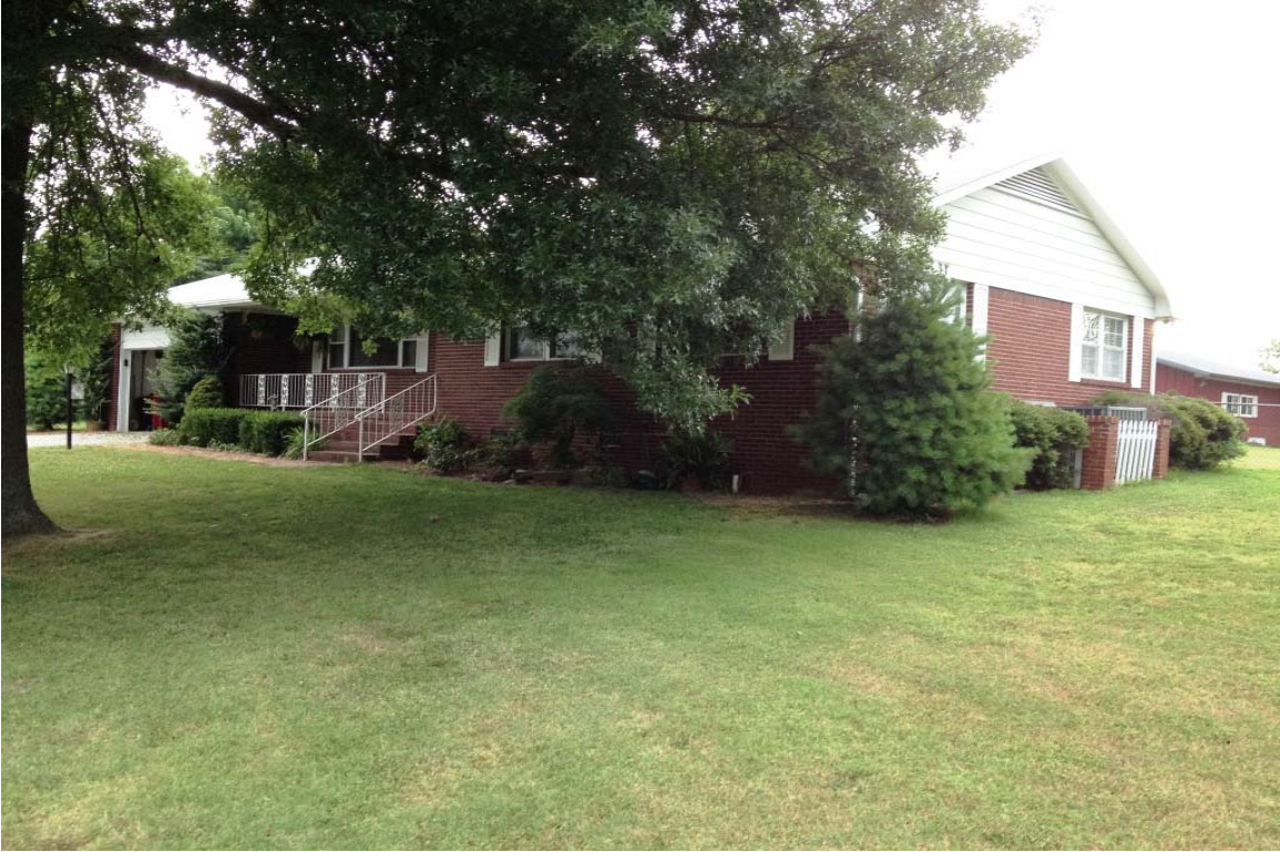
NORTHWESTERN AND SOUTHWESTERN ELEVATIONS OF 2648 OLD WIRE ROAD LOOKING NORTHERLY
