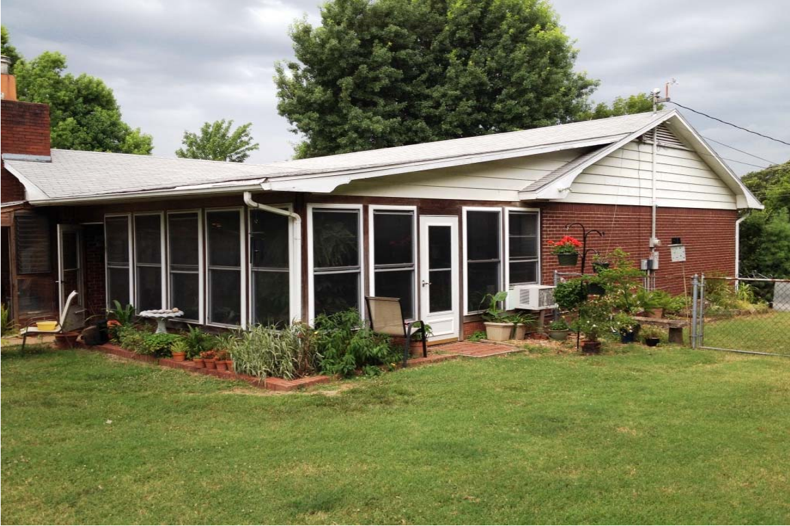
NORTHWESTERN AND SOUTHWESTERN ELEVATIONS OF 2648 OLD WIRE ROAD LOOKING SOUTHWESTERLY
