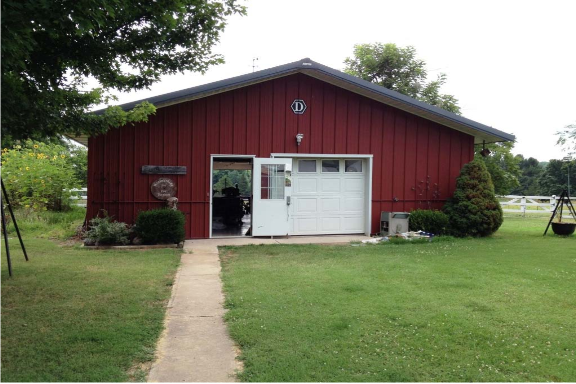
NORTHWESTERN ELEVATION OF SHOP BUILDING LOOKING SOUTHEASTERLY
