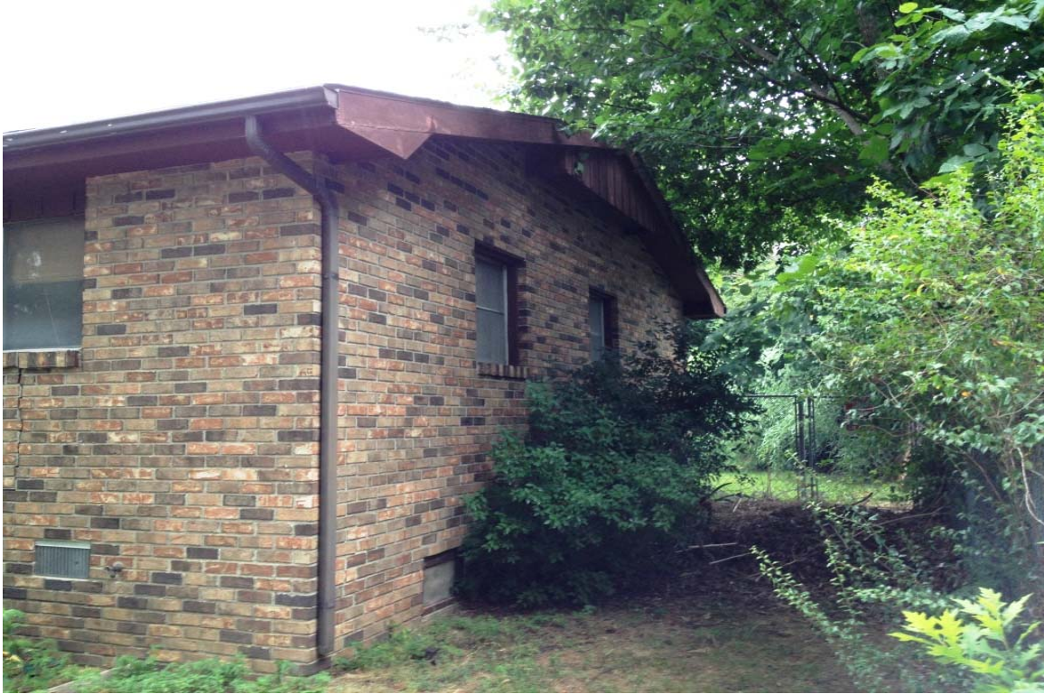
SOUTHWESTERN ELEVATION OF 2634 OLD WIRE ROAD LOOKING EASTERLY
