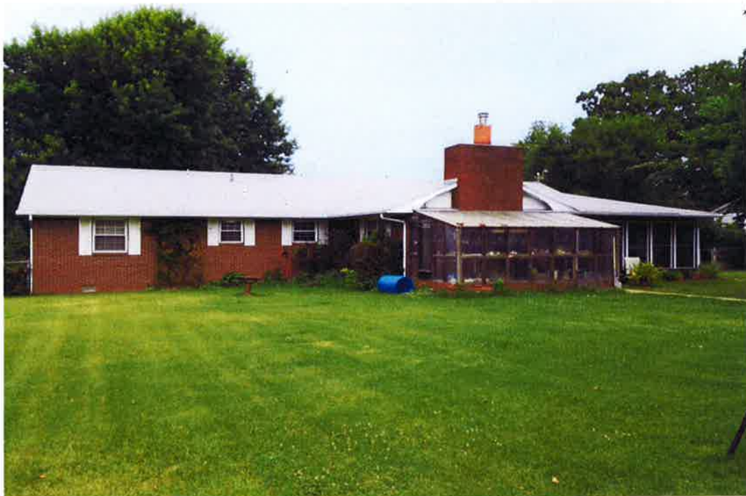
SOUTHEASTERN ELEVATION OF 2648 OLD WIRE ROAD LOOKING NORTHWESTERLY
