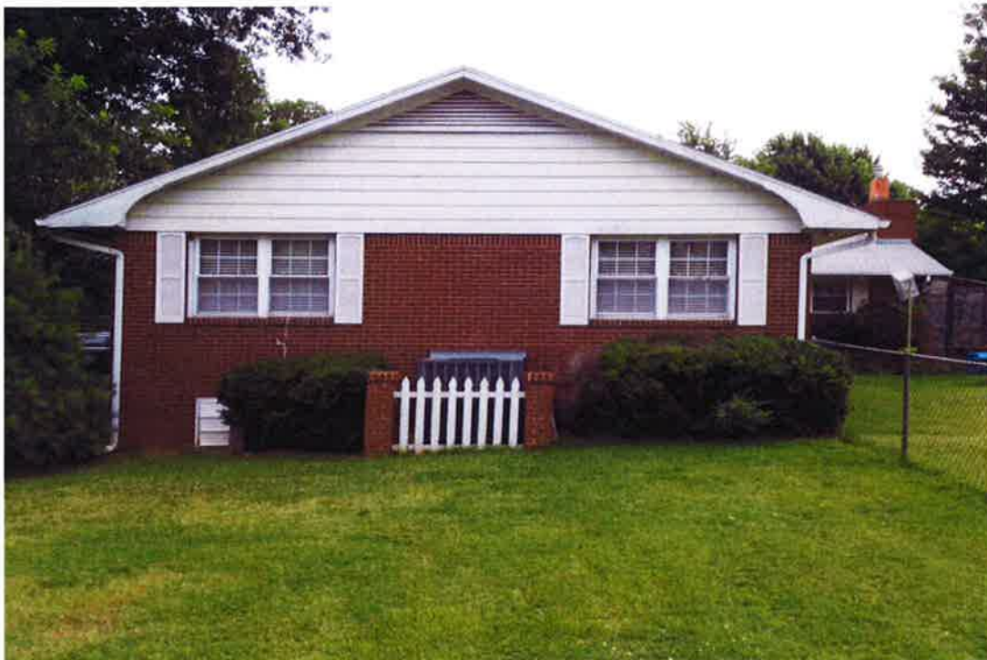
SOUTHWESTERN ELEVATION OF 2648 OLD WIRE ROAD LOOKING NORTHEASTERLY
