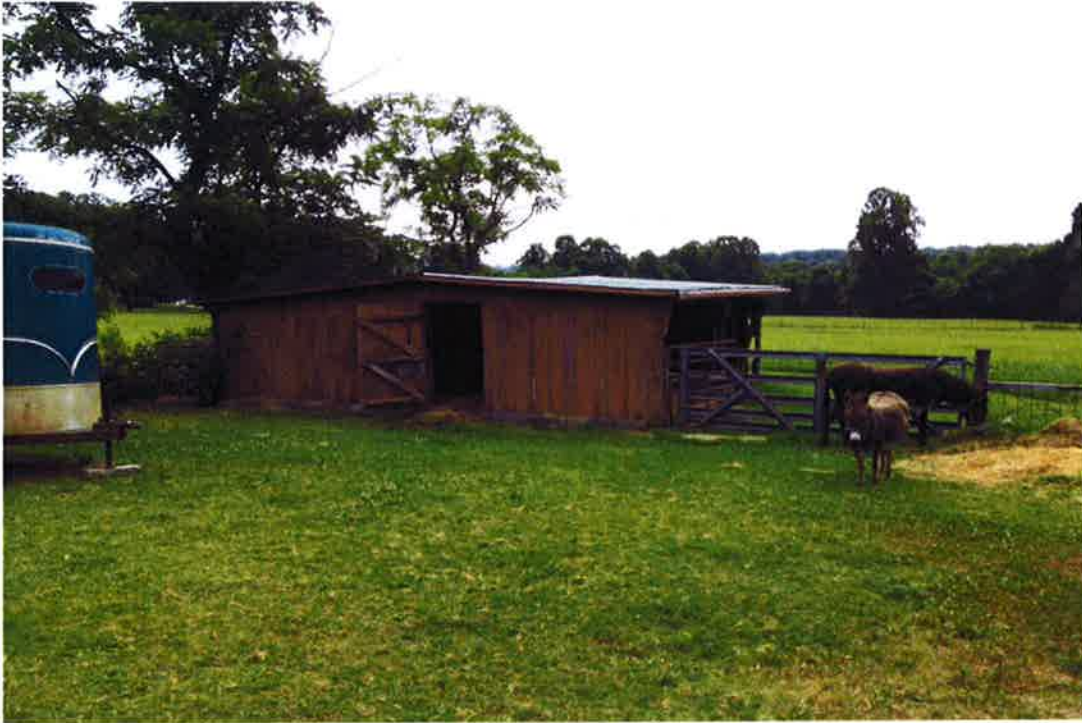
VIEW OF SHED AT 2648 OLD WIRE ROAD
