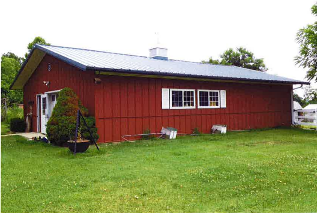
NORTHWESTERN AND SOUTHWESTERN ELEVATIONS OF SHOP BUILDING LOOKING NORTHERLY
