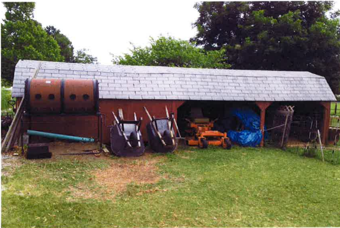
VIEW OF SHED AT 2648 OLD WIRE ROAD
