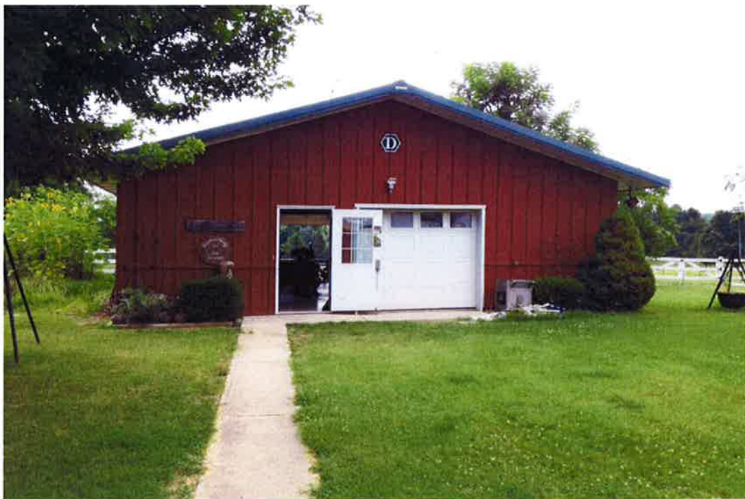
NORTHWESTERN ELEVATION OF SHOP BUILDING LOOKING SOUTHEASTERLY
