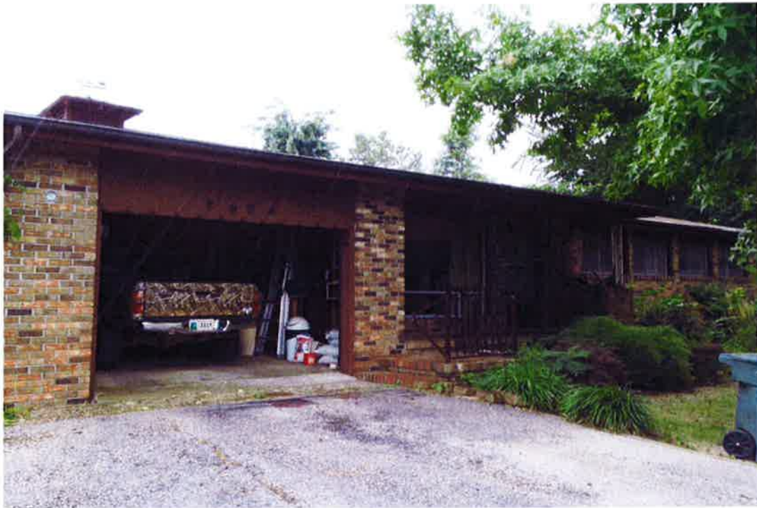
NORTHWESTERN ELEVATION OF 2634 OLD WIRE ROAD LOOKING SOUTHERLY
