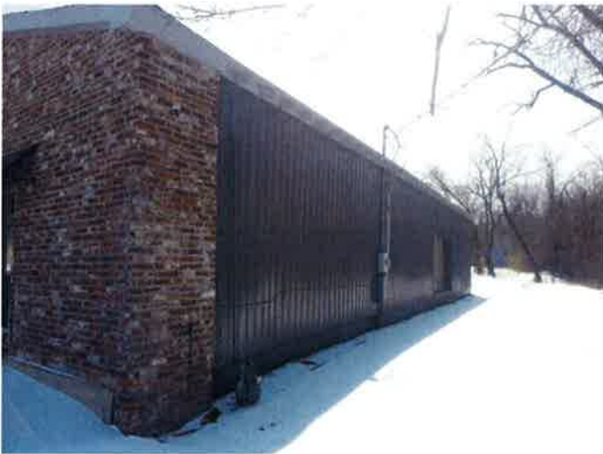
Side View of Building (West side) at 701 W North St.
