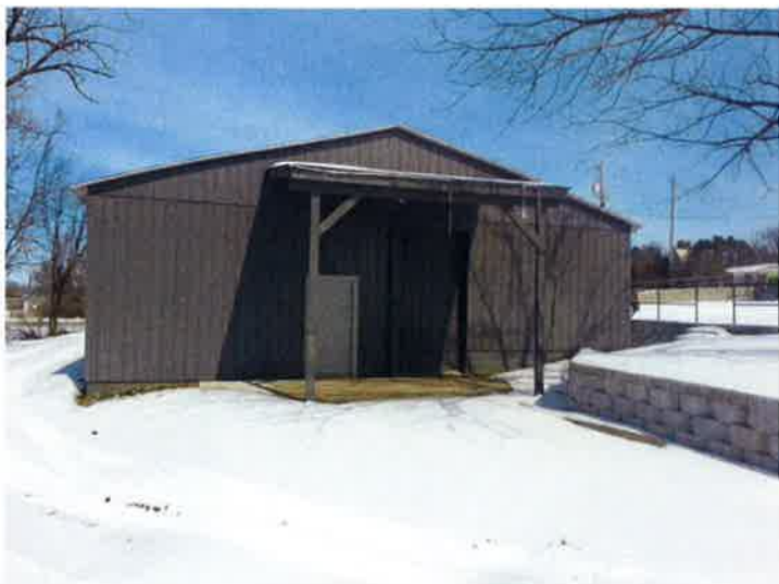
Rear View of Building at 701 W North St.
