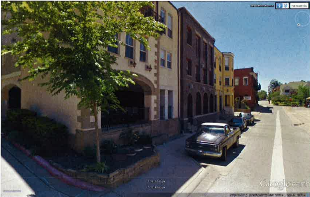
The Three Sisters building on Dickson Street successfully blends the first floor parking deck with the residential and commercial portions of the development using similar materials and detailing throughout the project.
