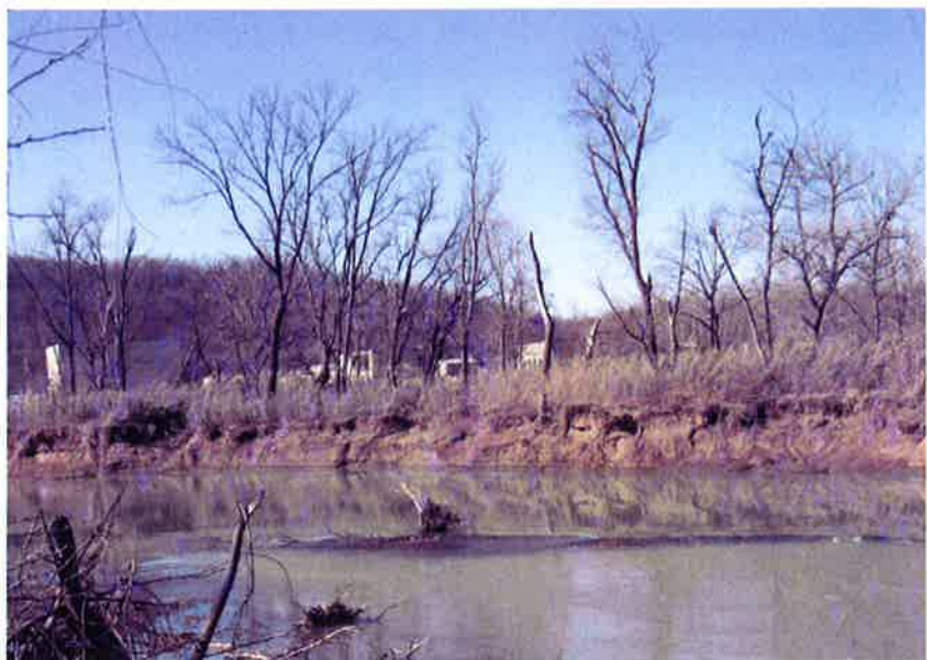
Figure 2 Eroding river bank near Noland Waste Water Treatment Plant
