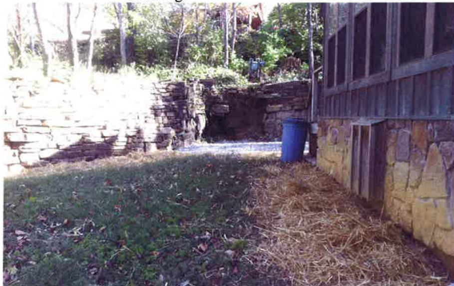
Damaged and Undamaged Wall Sections
