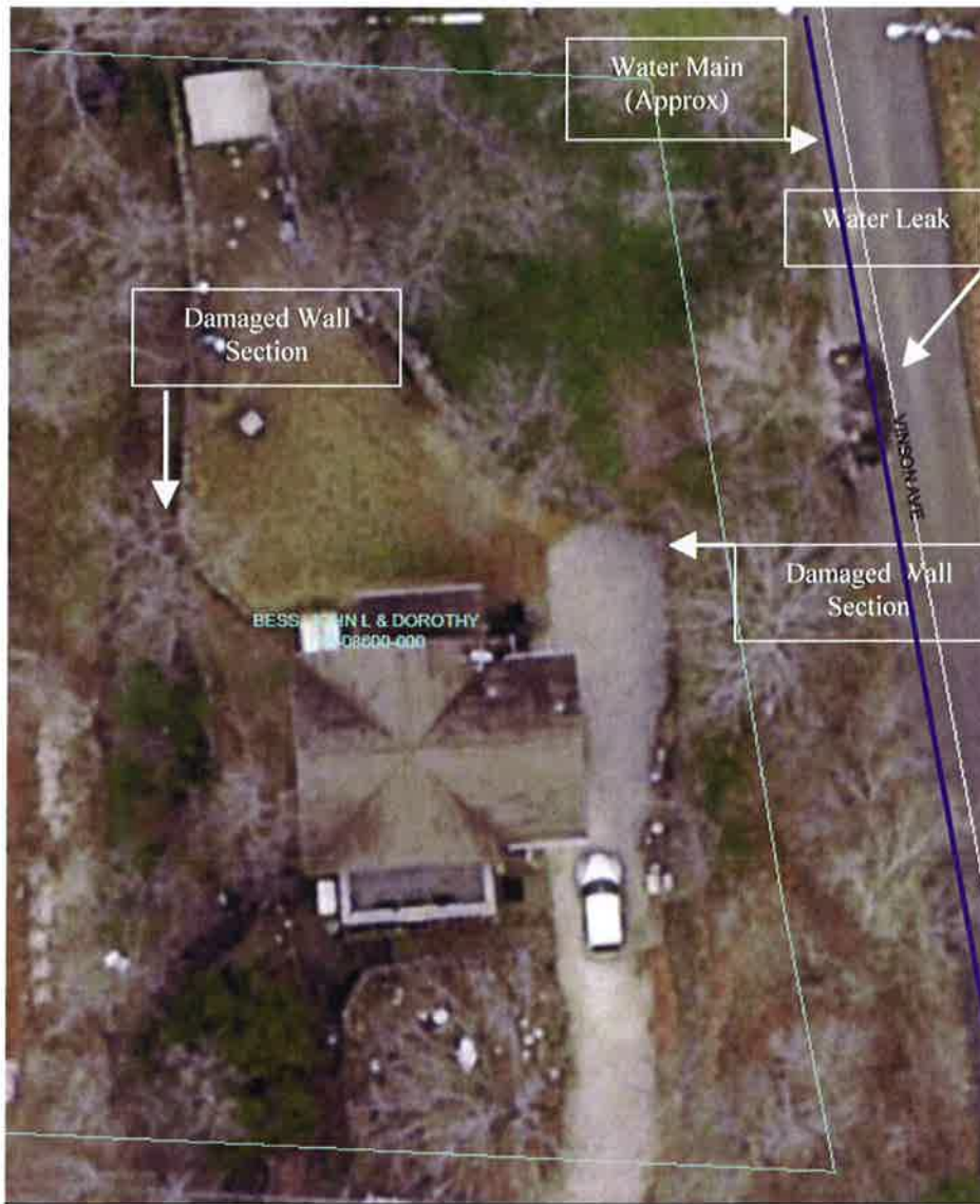
Aerial Photo Showing Relative Locations of Wall and Leak
