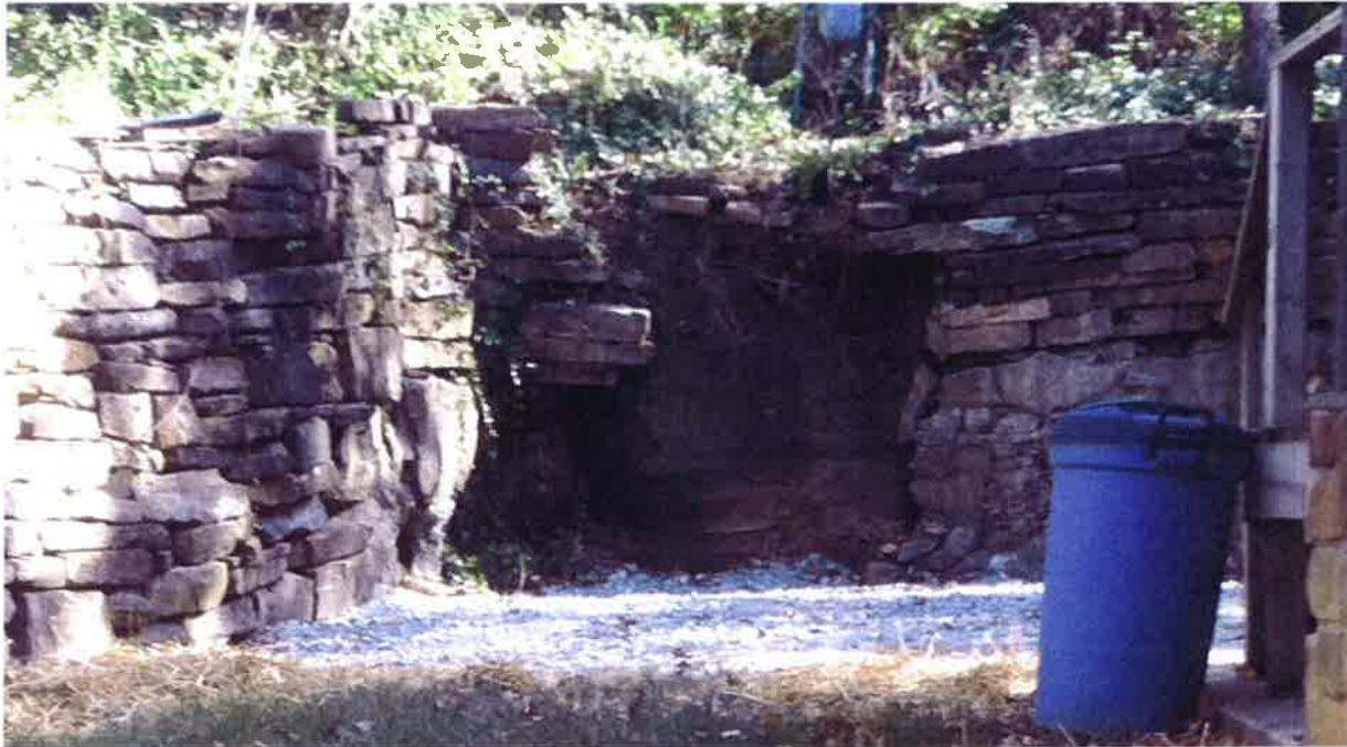
Close-up of Damaged Wall Section
