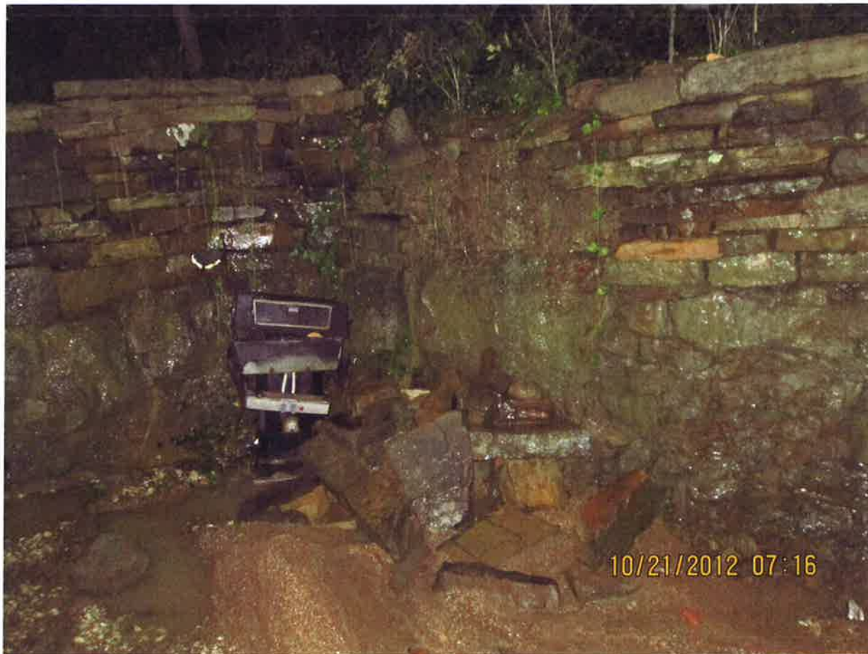
Damaged Wall Section the Morning of the Leak
